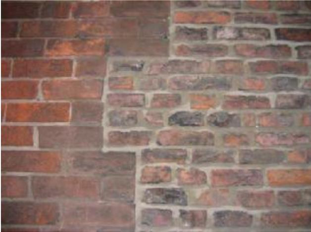
Fig: 1 The join between the front of 14 to 18 High Street and the side. The difference in brick sizes is very clear, indicating this is not just a different style of bricklaying (which is popular in many houses in the area) but a different phase of building.
