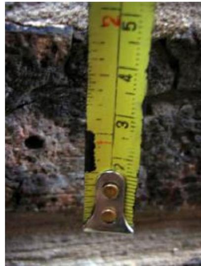
Fig: 2 This image shows clearly the size of the bricks running down the side of the building (inches to the left and centimetres to the right). Bricks of this size indicate an early build.
